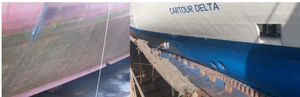
Image 11. Coating refitting of the hull of M/V Cartour Delta, owned by Caronte & Tourist shipping company (Bluetech.eu, 2016).
