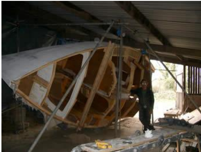
Sam Watt's CR25 All planked and in the process of being turned up right ready for fitting out.
