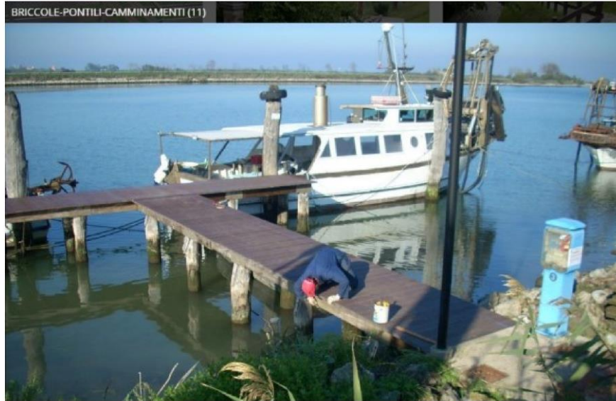
Image 20. A pier made from PRECO SYSTEM with recycled plastic boards (BlueTech.eu, 2016)
